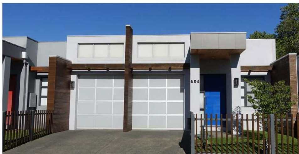
Figure 5 Example of semi-detached dwelling (604 Olive Street, Albury)
